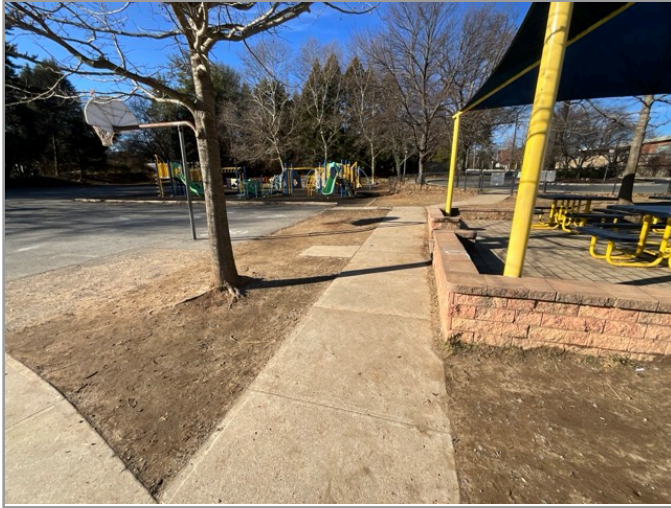
ACCESSIBLE ROUTE TO PLAYGROUND
