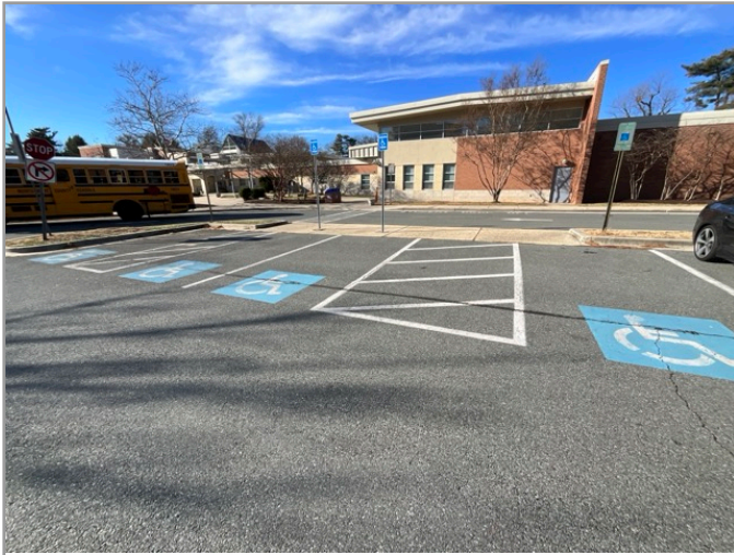
OVERVIEW OF ACCESSIBLE PARKING AREA
