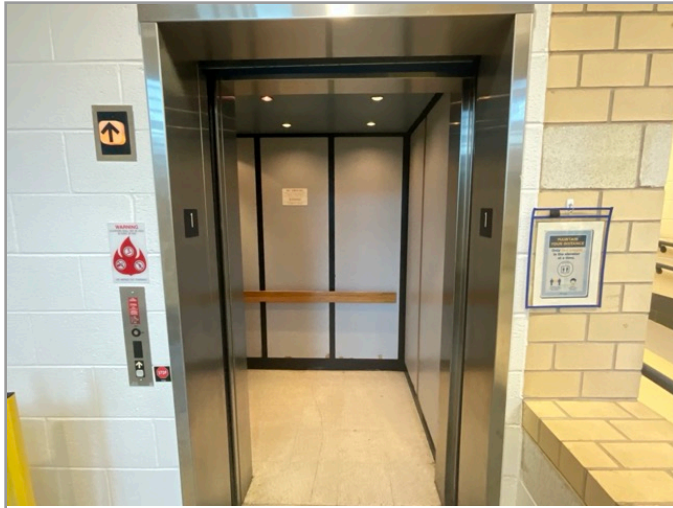
LOBBY LOOKING AT CABS
